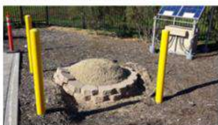
Figure 3. Subsidence at EOCG. Note the seismic vault has clearly subsided, and the yellow posts have been recently installed. Photo courtesy of Dan Deleman, USGS. Photo taken on January 6, 2015.
